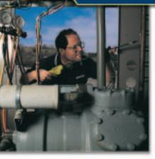
The Informant™2 leak detector allows pinpoint detection of both refrigerant and combustible gas leaks with the same instrument.
